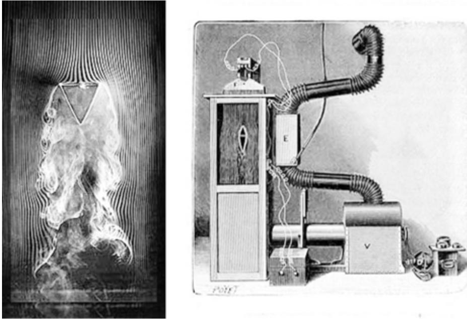
**Fig. 2.9.** A typical Marey's image of coherent structures (a) observed in his wind tunnel (b), published in 1901.
